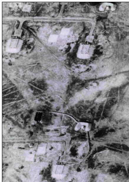
Exposed? A VA panel says nerve gas in Iraq’s Khamisiyah weapons depot, shown here after it was demolished, likely contributed to Gulf War illness.
